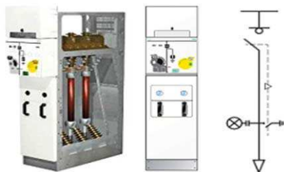
Figure 2. Fluokit M24+ switch disconnector [15].
