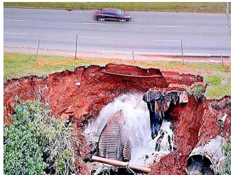
Figure 2. Major erosion resulting from a broken water pipeline in Brazil.
