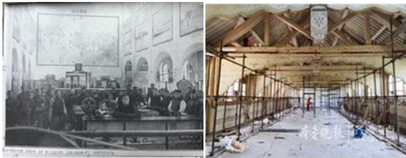
Figure 12. Interior of the museum. With no need for extra support inside the Chinese-style wooden structure, the wooden pillars and arches become a kind of subjective decoration. The left from Angus Library, The BMS archive records, property in China . right from Qilu Newspaper , 18 May 2018.
