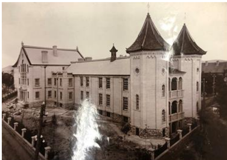
Figure 29. The west and north façades of Jinan Hospital, 1916, property in China. Photo from Oxford University, Angus Library, The BMS archive records, , property in China .
