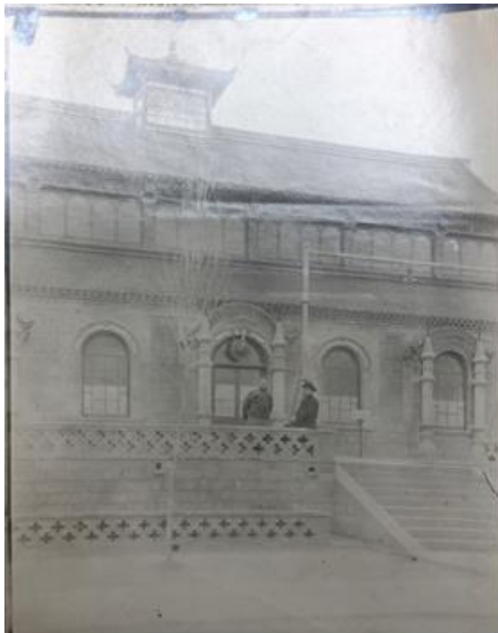
Figure 1. The Jinan museum, 1906. The museum had already become a group of buildings organized around a walled garden . However, the schools mentioned in the record had not yet appeared. The man on the right is J.S. Whitewright. Photo from Oxford University, Angus Library, The BMS archive records, , property in China .
