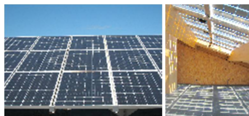
Figure 3: Integrated PV roof panel (left: external view, right: internal view)
