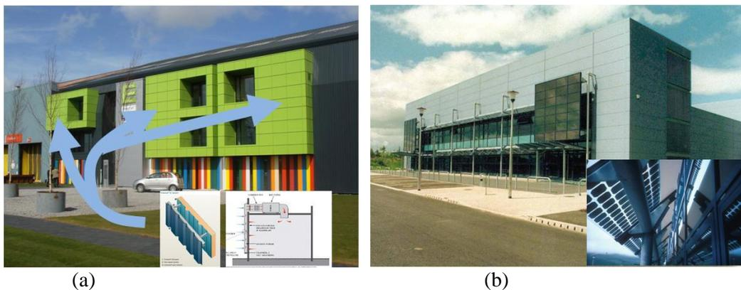
Figure 7. (a) Transpired solar collectors (TSC's) for collecting thermal energy through south facing cladding systems for solar air heating. (b) PV system used as shading device.
