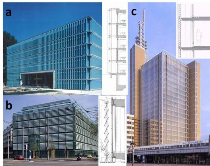
Figure 3. Adjustable external blind systems in (a) EMPA, (b) Ta-Media offices in Zurich, and (c) Hannover EXPO HQ.
